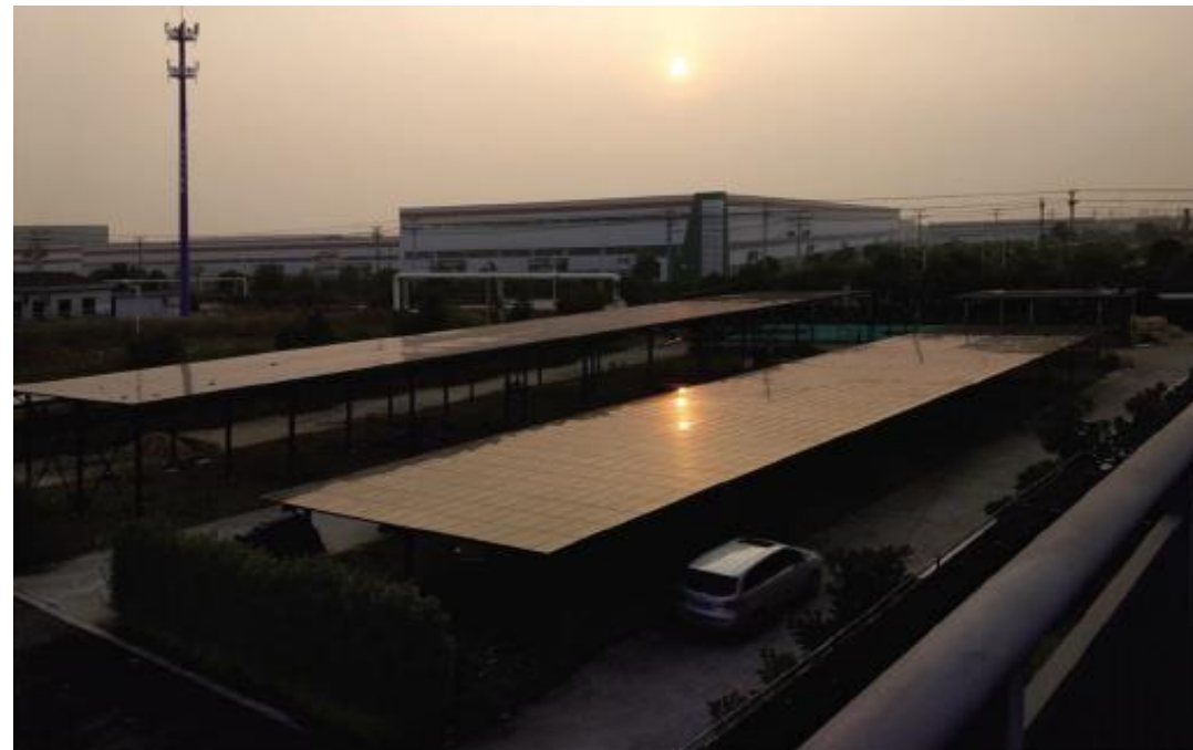
光伏车棚 Photovoltaic Vehicle shed
