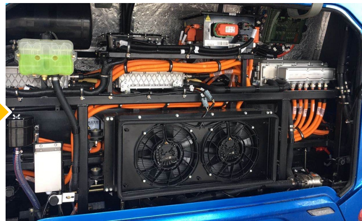
EV Cooling System
